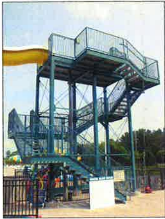
INSTALL NEW ANCHOR RODS AT EXIST'G COLUMNS
