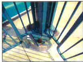
CUT EXIST'G CORRODED ANCHOR RODS
